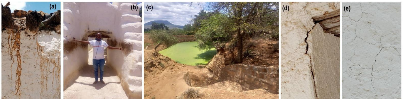
Figure 7. (a) Drainage marks on the walls of shrine. (b) Staining in places where worshippers kiss the walls of the shrine or rub their hands on it, sometimes with butter and blood which changes the colour. (c) Haro Luku pond built by Sheikh Hussein in the 10th century containing holy water (Zamzama), used only for drinking purposes. (d) Cracked pillar in the shrine, probably because of rain entering from the roof (e) Crazed walls of the shrine. Photographs by author H.G.T., August 2022.
